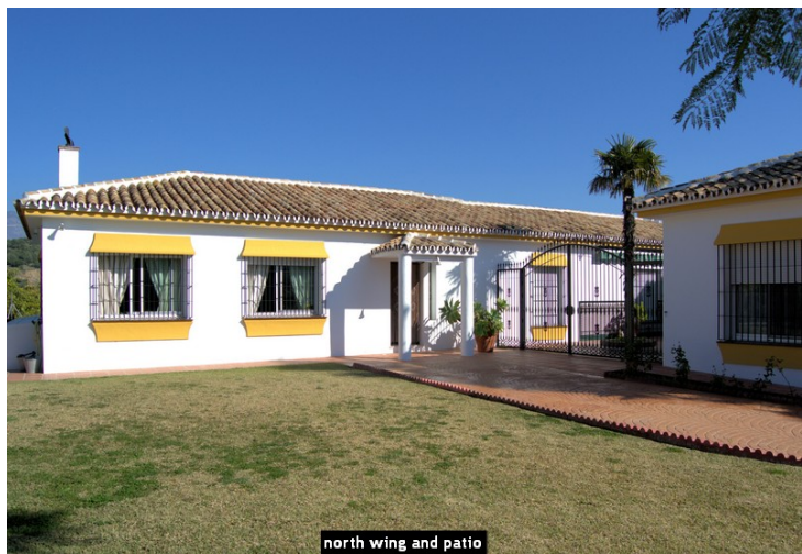
north wing and patio
